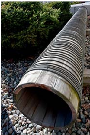
Stuart Issett for The New York Times An unused wood water pipe kept at the Public Works office in Chelan, Wash.
