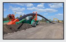
The spider plow can install HDPE pipe up to 24" dia. to a depth of 6'. It saves water utilities big dollars on main replacement and new installations.
