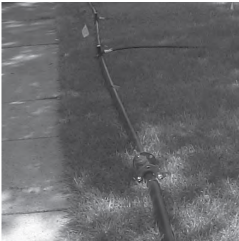
Figure 19 Example of Above Ground PE Bypass Pipe
