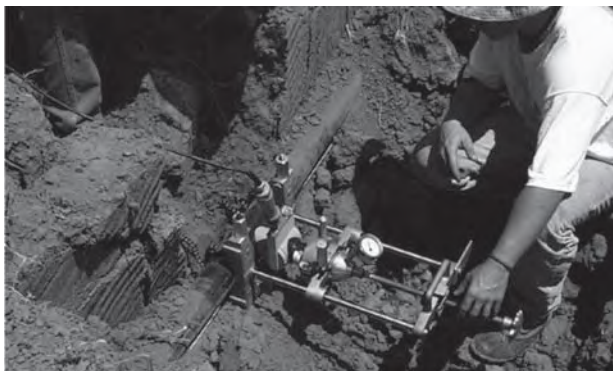
Figure 3 Saddle Fusion Repair
