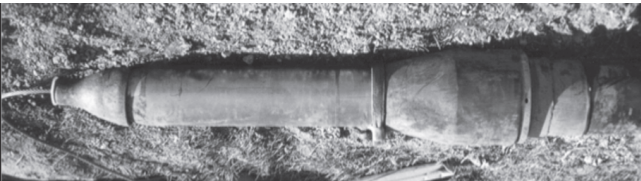
Figure 2 The Bursting Head of the Pneumatic System
