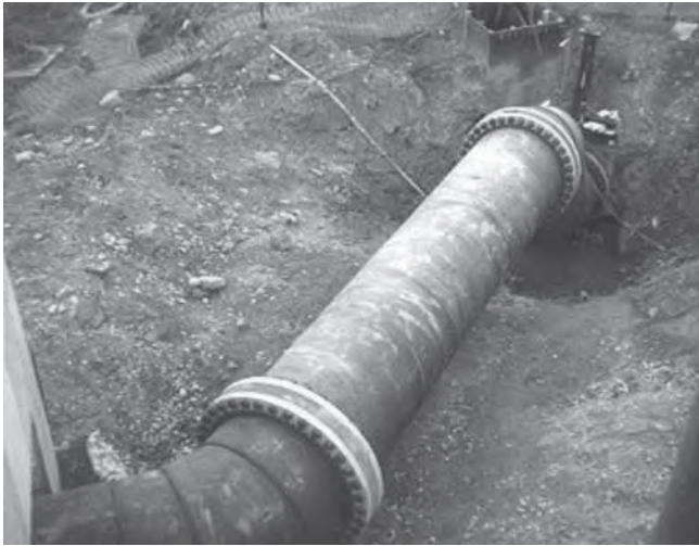
Figure 13 Flange Adapter Assembly
