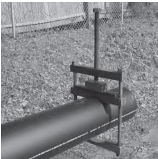
Figure 15 Mechanical Re-Rounding Clamp Installed
