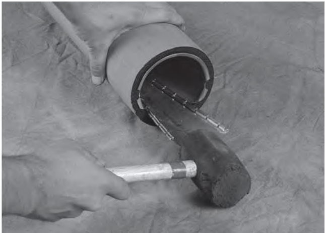
Figure 12 Install Split Ring Stiffener in PE Pipe
