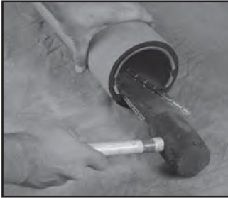
Figure 19 Install Split Ring Stiffener in PE pipe
