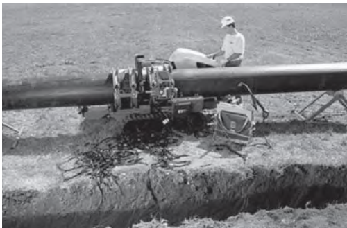
Figure 1 Above Ground Repair with Fusion Machine
