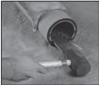
Figure 19 Install Split Ring Stiffener in PE pipe
