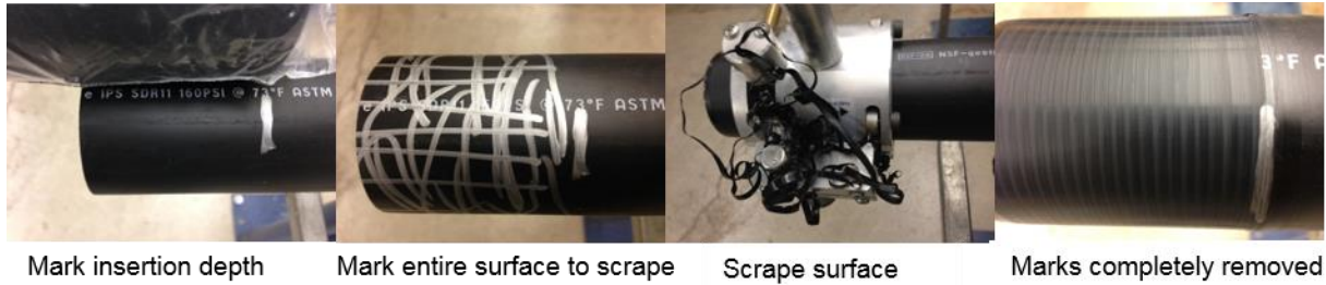
Figure X-o - Correct Scraping
