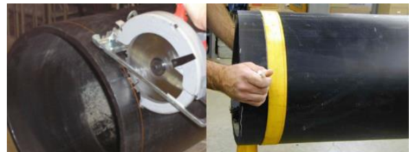
Figure IV-d – Marking and cutting larger diameter pipes
