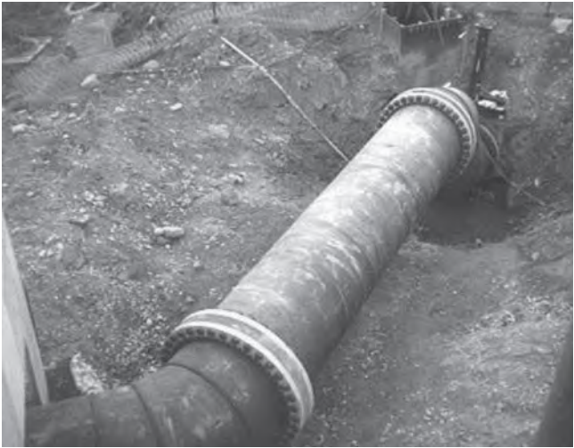
Figure 13 Flange Adapter Assembly
