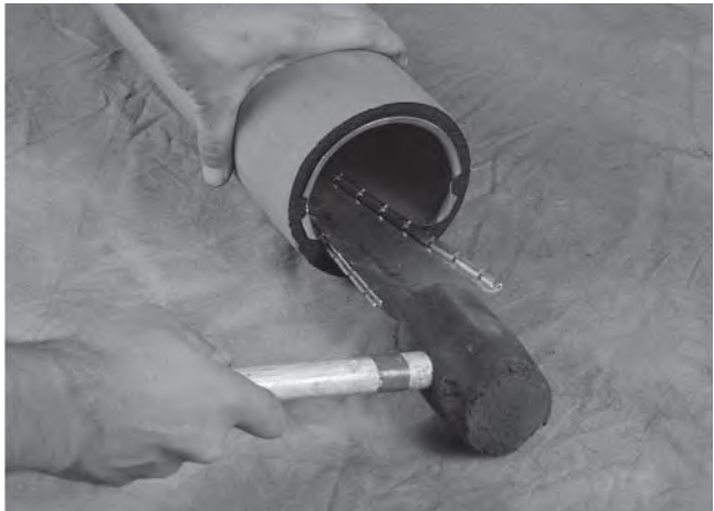
Figure 12 Install Split Ring Stiffener in PE Pipe
